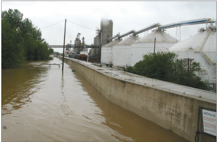
FLOODWALL DURING THE MISSISSIPPI RIVER FLOOD OF 2011 IN THE MEMPHIS DISTRICT (SOURCE: USACE).
