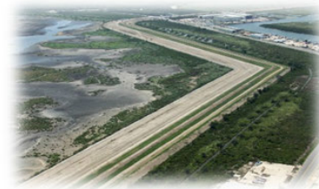
Image: Typical Earthen Levee in USACE Inventory
