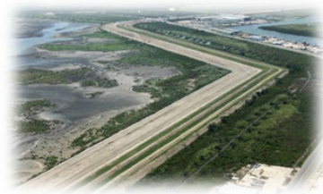
Image: Earthen Levee in Inventory
