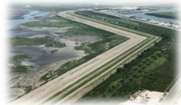
Image: Earthen Levee in Inventory
