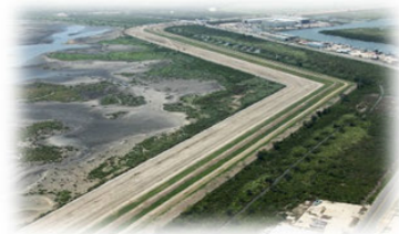
Image: Earthen Levee in Inventory
