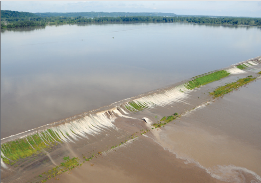
OVERTOPPING OF THE L-550 LEVEE IN ATCHISON COUNTY, MISSOURI, DURING A MISSOURI RIVER FLOOD, JUNE 2011 (SOURCE: USACE).
