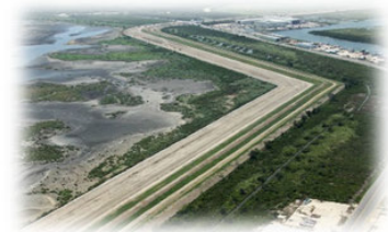
Image: Earthen Levee in inventory
