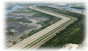
Image: Earthen Levee in Inventory
