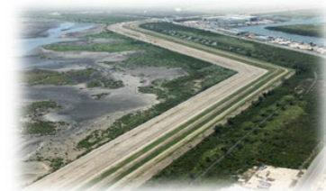
Image: Earthen Levee in Inventory
