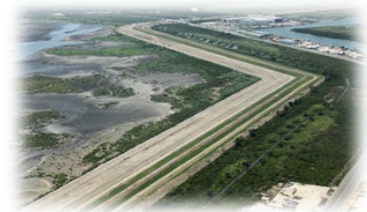
Image: Earthen Levee in Inventory
