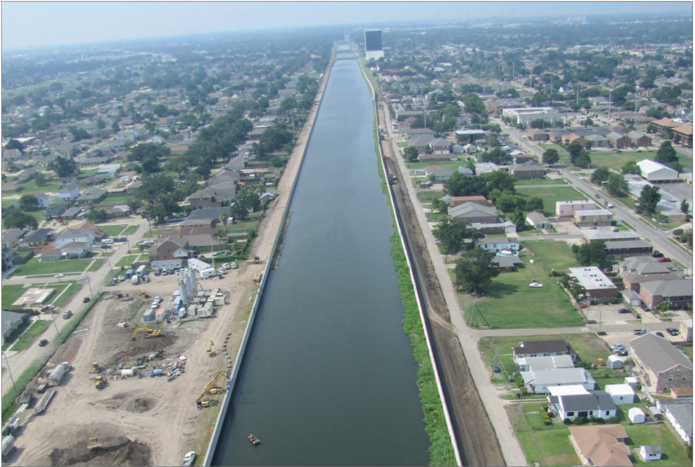
I-WALLS ALONG THE 17TH ST. CANAL IN NEW ORLEANS (SOURCE: USACE).
