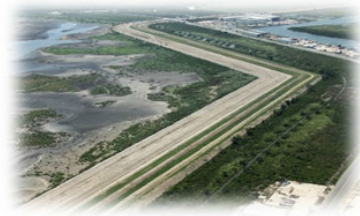
Image: Earthen Levee in Inventory
