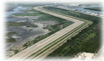
Image: Earthen Levee in Inventory
