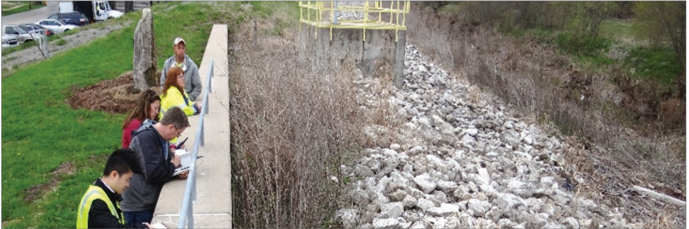
USACE STAFF AND THE NON-FEDERAL SPONSOR CONDUCTING A LEVEE INSPECTION IN ST. PETERS, MISSOURI (SOURCE: USACE).
