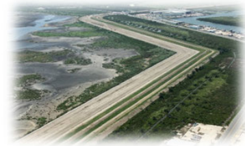
Image: Earthen Levee in Inventory
