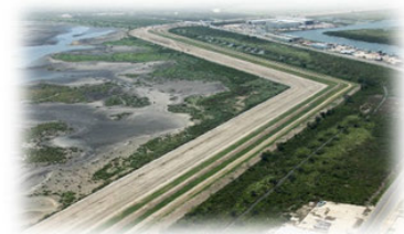
Image: Earthen Levee in Inventory
