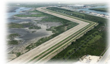
Image: Earthen Levee in Inventory
