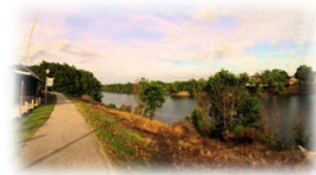
Image: Northport Levee Protected Area Tuscaloosa, Alabama
