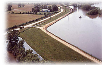
Image: Winona Levee Winona, Minnesota
