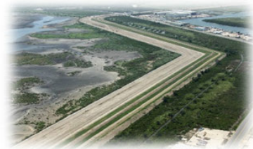
Image: Earthen Levee in Inventory
