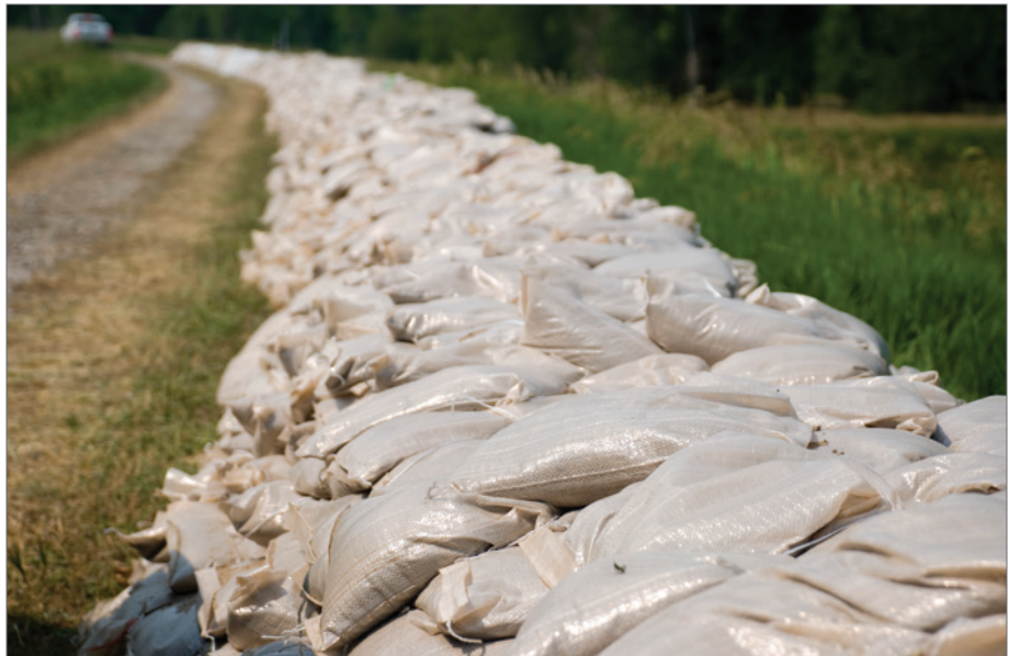
SANDBAGS PLACED ON TOP OF A LEVEE NEAR FOREST, MISSOURI, DUE TO OVERTOPPING CONCERNS FROM A RISING MISSOURI RIVER IN JUNE 2011 (SOURCE: USACE).
