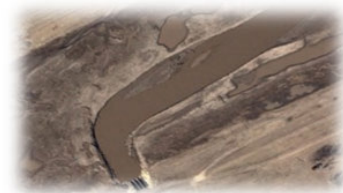
Image: Wichita Levee Wichita, Kansas
