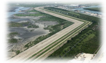
Image: Embankment Levee in Inventory
