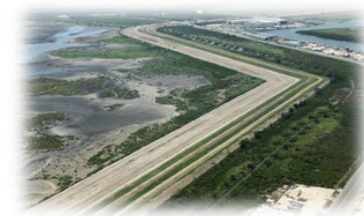
Image: Earthen Levee in Inventory
