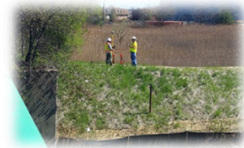
Image: Elizabeth River Right Bank Levee Elizabeth, New Jersey
