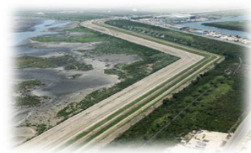
Image: Earthen Levee in Inventory
