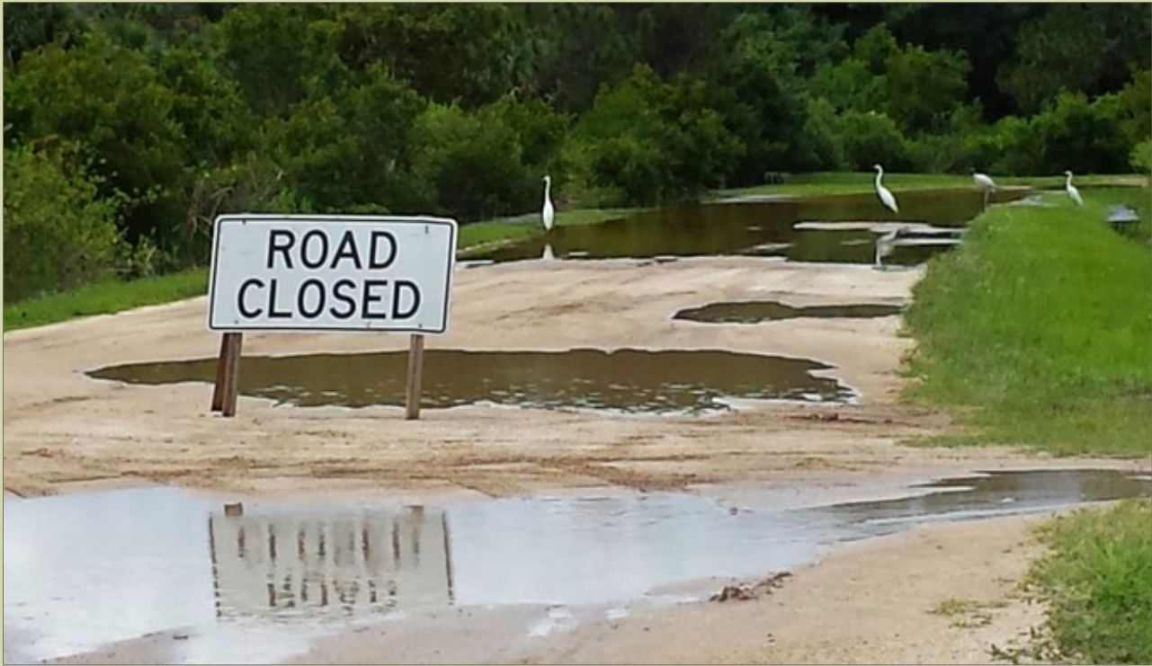
A FLOODED ROADWAY (SOURCE: ISTOCK).
