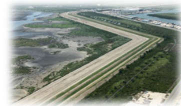
Image: Earthen Levee in Inventory
