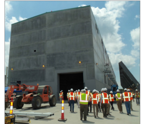
GULF INTRACOASTAL WATERWAY (GIWW) WEST CLOSURE COMPLEX PUMP STATION IN NEW ORLEANS, LOUISIANA, MAY 2011 (SOURCE: USACE).
