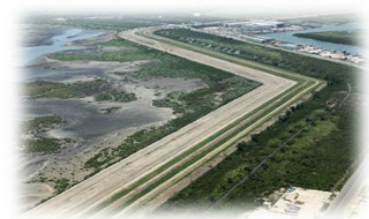
Image: Earthen Levee in Inventory
