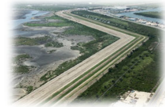
Image: Embankment Levee in Inventory
