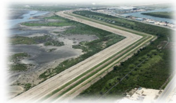
Image: Earthen Levee in Inventory
