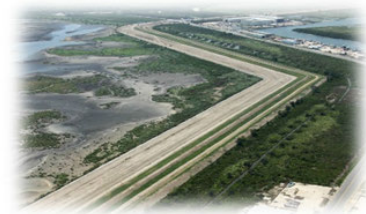
Image: Earthen Levee in Inventory
