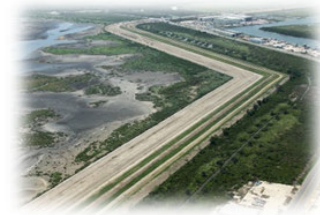
Image: Embankment Levee in Inventory
