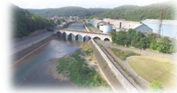
Image: Cumberland Levee Cumberland, Maryland
