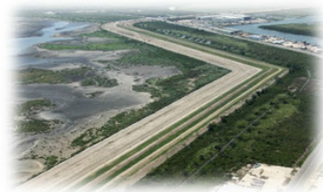
Image: Earthen Levee in Inventory
