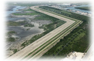
Image: Embankment Levee in Inventory
