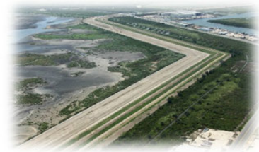
Image: Earthen Levee in Inventory
