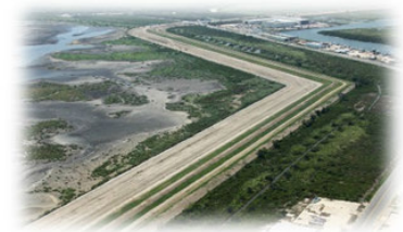
Image: Earthen Levee in Inventory
