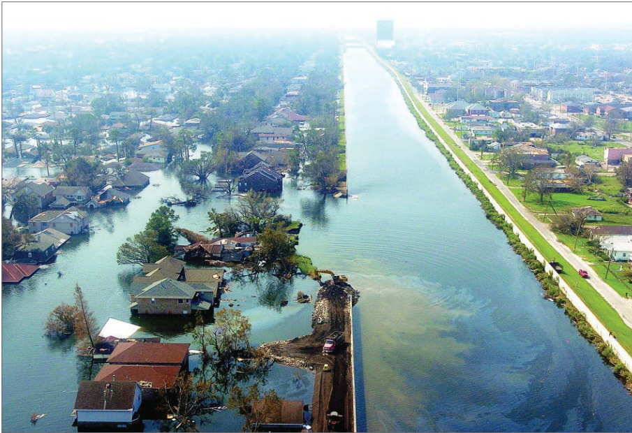
17TH STREET CANAL LEVEE BREACH IN NEW ORLEANS, LA, SEPTEMBER 3, 2005 (SOURCE: BRETT DUKE, THE TIMES-PICAYUNE ARCHIVE).
