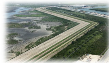
Image: Earthen Levee in Inventory
