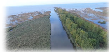
Image: Sebewaing River Levee, Sebewaing, Michigan
