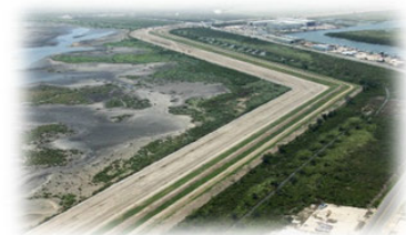
Image: Earthen Levee in Inventory
