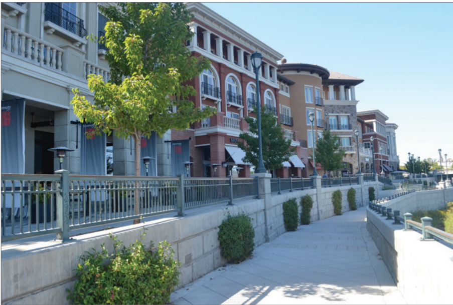
A VIEW OF THE TERRACED FLOODWALL THAT ALSO SERVES AS WALKING PATH ALONG THE NAPA RIVER, CALIFORNIA (SOURCE: USACE/DEDE CORDELL, HTTPS://FLC.KR/P/AQWPUG ).
