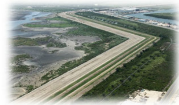
Image: Earthen Levee in Inventory
