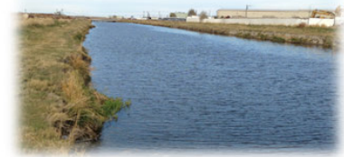
Image: Surplus Canal Levee, Salt Lake City, Utah
