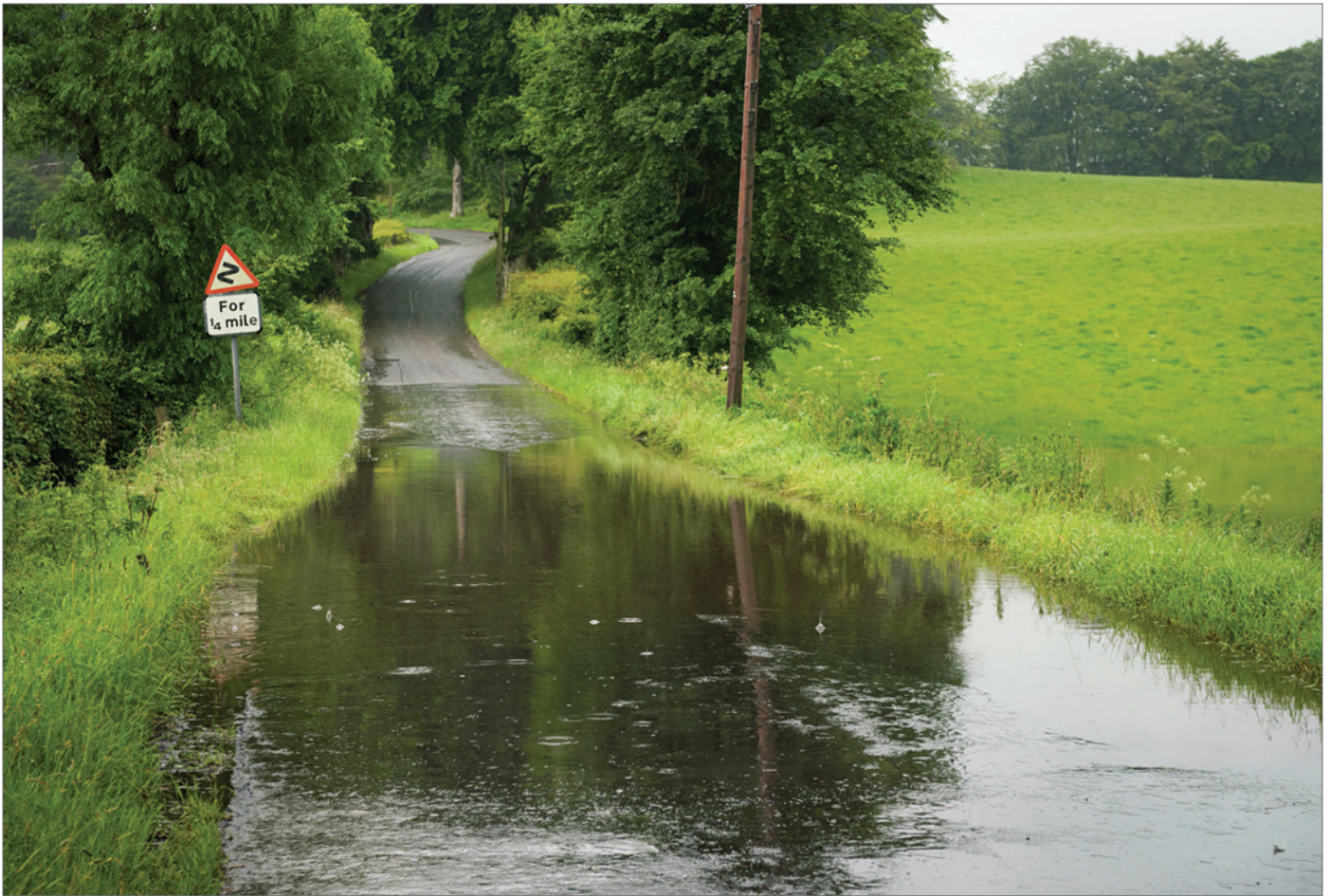
A FLOODED ROADWAY (SOURCE: ISTOCK).
