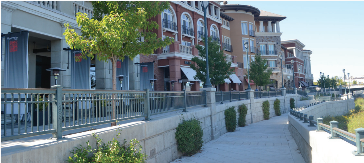
A VIEW OF THE TERRACED FLOODWALL THAT ALSO SERVES AS WALKING PATH ALONG THE NAPA RIVER, CALIFORNIA (SOURCE: USACE/DEDE CORDELL, HTTPS://FLIC.KR/P/AQWPUG ).
