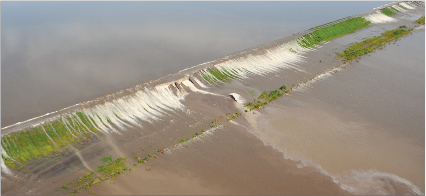
OVERTOPPING OF THE L-550 LEVEE IN ATCHISON COUNTY, MISSOURI DURING A MISSOURI RIVER FLOOD, JUNE 2011 (SOURCE: USACE).
